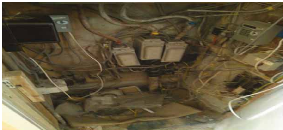
Figure 4. Open sockets and wires in asylum seeker house where children are living
