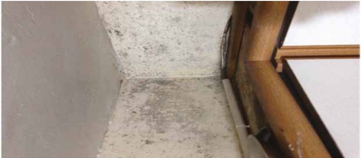
Figure 2. Damp in bathroom in an asylum seeker house in Belfast
